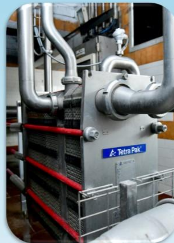
Regenerative Heat Exchanger
